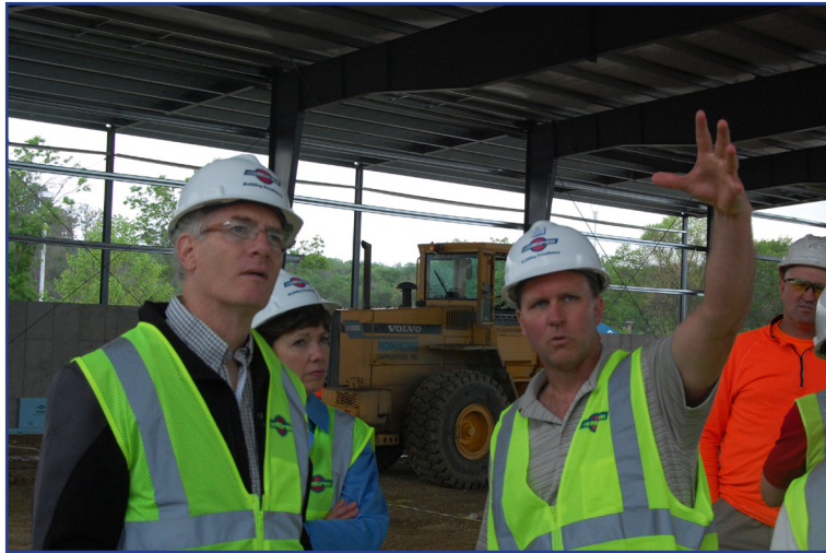
Left: Mark Clarke, AEC General Manager, shows George and Debbie Crave the construction progress.
