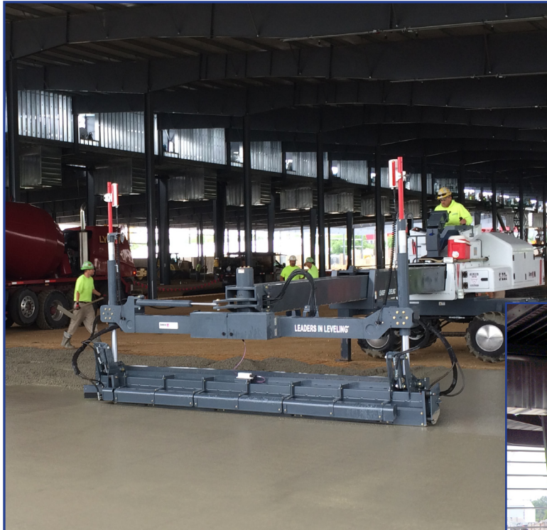
Left and Below: The floor in Pavilion 2
