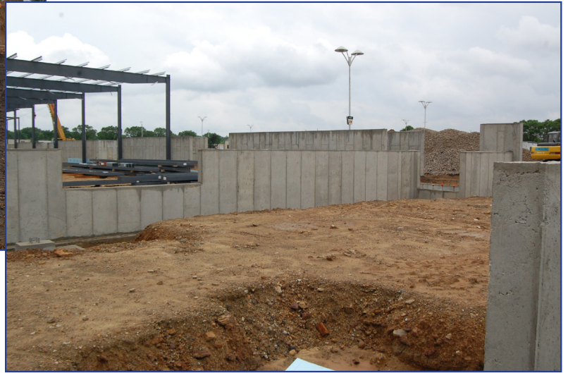
Left and Below: The outside entrance into the milking parlor and what will become the finished parlor space.
