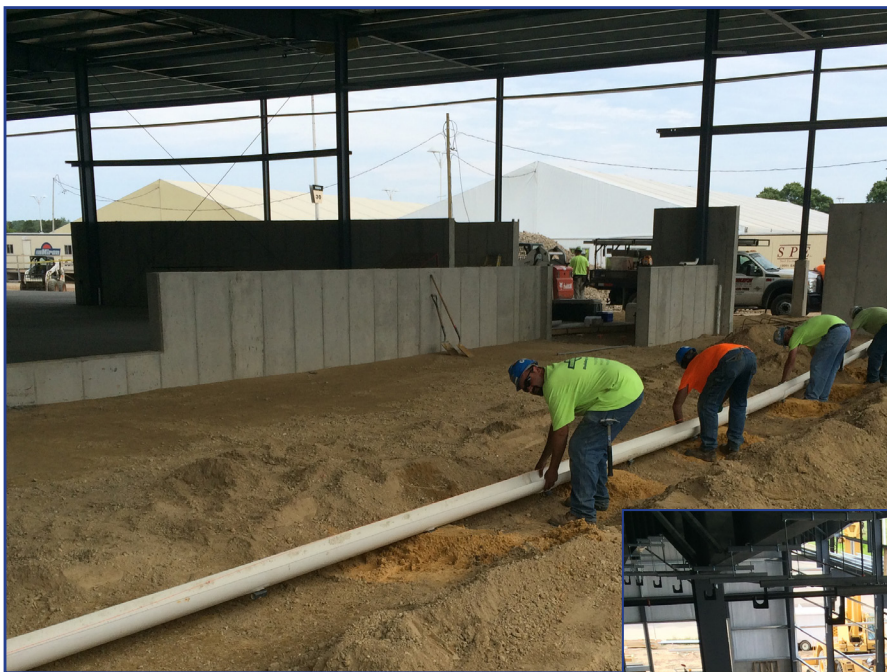
Left: Laying the floor drain for the parlor
