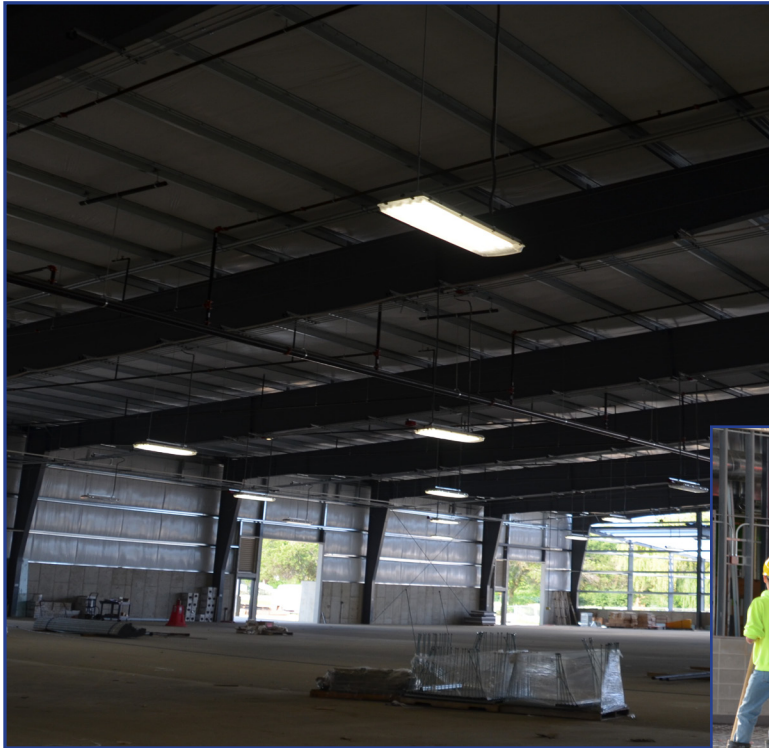
Left: Energy efficient lights are being installed in Pavilion 2.
