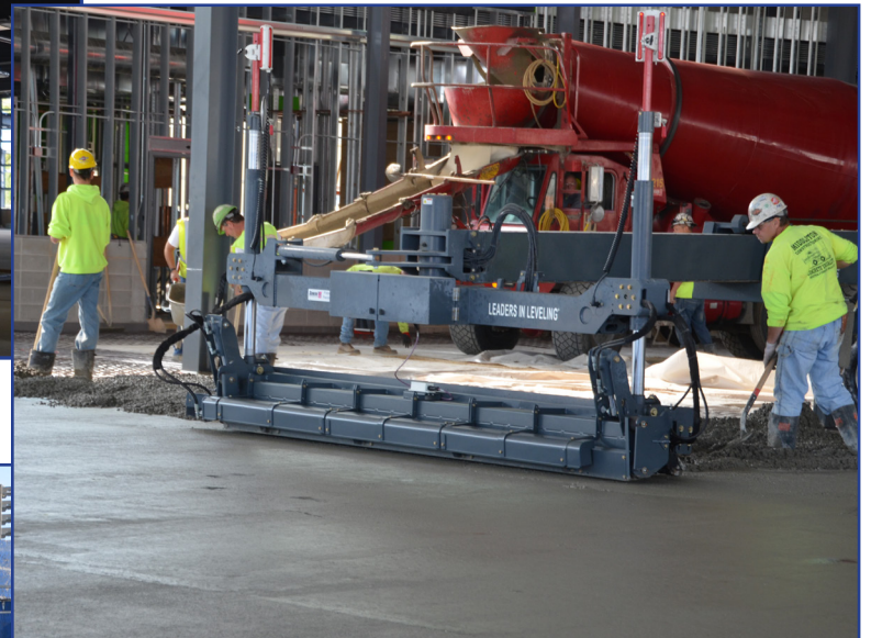
Below: Pouring the rest of the floor in Pavilion 1.
