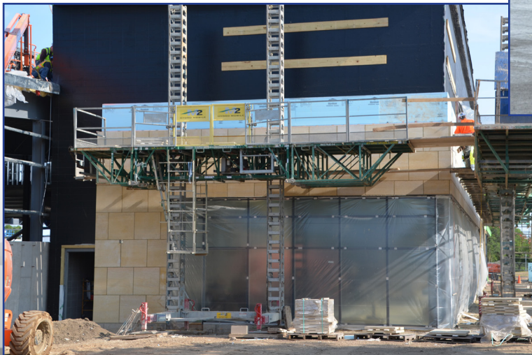
Left: The exterior on Pavilion 1 will have 68,000 pounds of block facing when completed.
