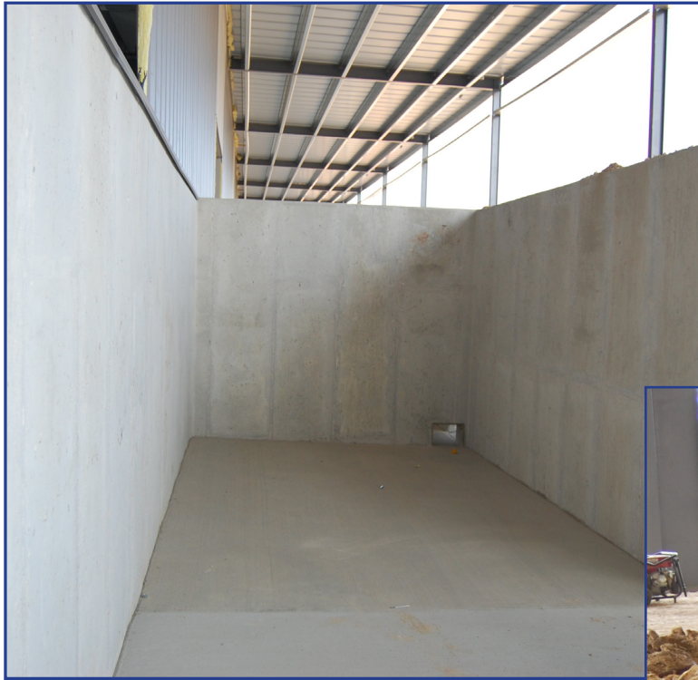
Left: Completed manure bunker.
