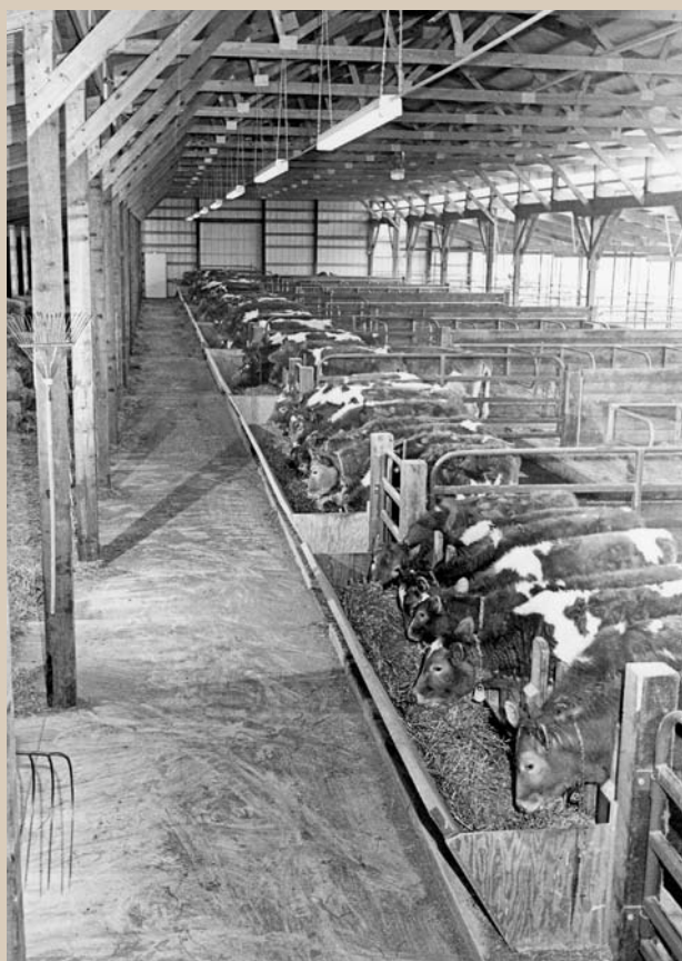
THIS 30-YEAR-OLD HEIFER BARN , 63 by 180 feet, was converted into a bedded pack, close-up facility by removing the free stalls.
