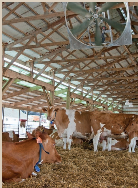
CLOSE-UPS WILL HAVE at least 100 square feet of bedded pack each, plus no less than 28 inches of bunk space per cow. The building's ventilation was improved by replacing north wall siding with curtains and adding fans. It remains open to the south. There are two calving pens with a head gate, plus a small, warm room with hot water and a freezer for storing colostrum.
